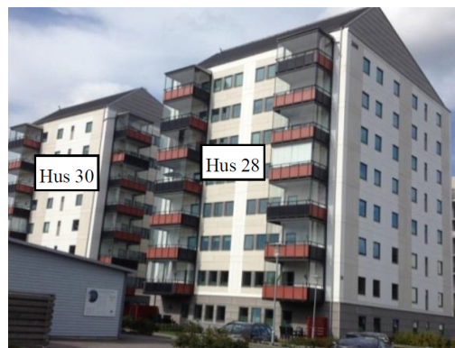
Figure 1. Two wood-framed passive houses in Portvakten Söder.
