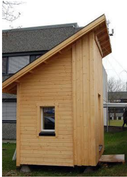
Figure 2. An image of the test building from the east direction.
