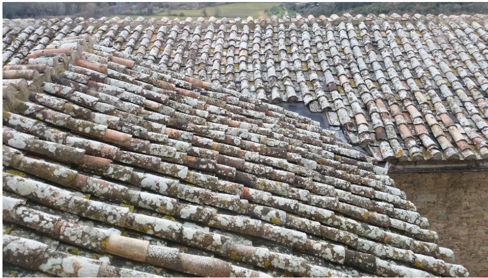
Figure 7. View of the case study's roof with the original tiles.
