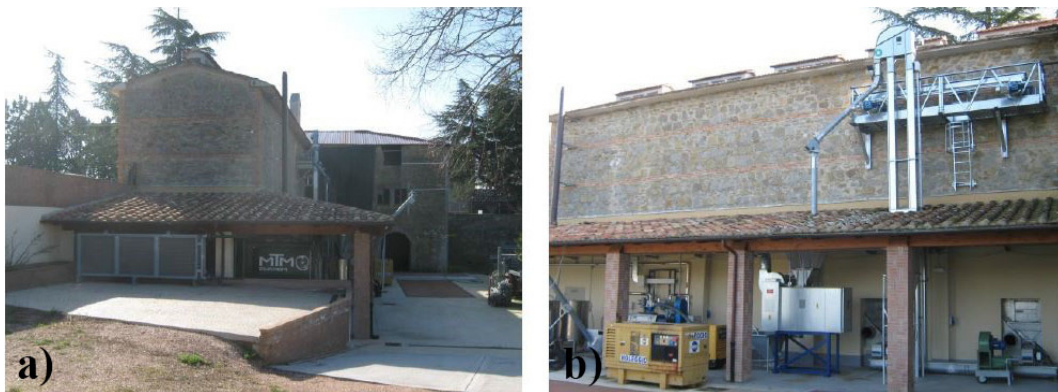
Figure 11. Side (a) and front (b) view of the installed pilot plant.
