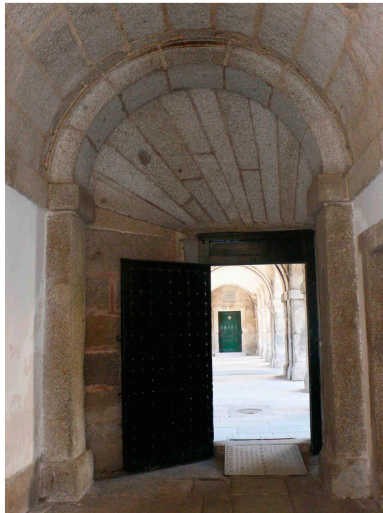
Figure 18. Arcade to the Compañía as seen from the Botica. The stereotomy of the vault must be stressed. Photograph by the authors.
