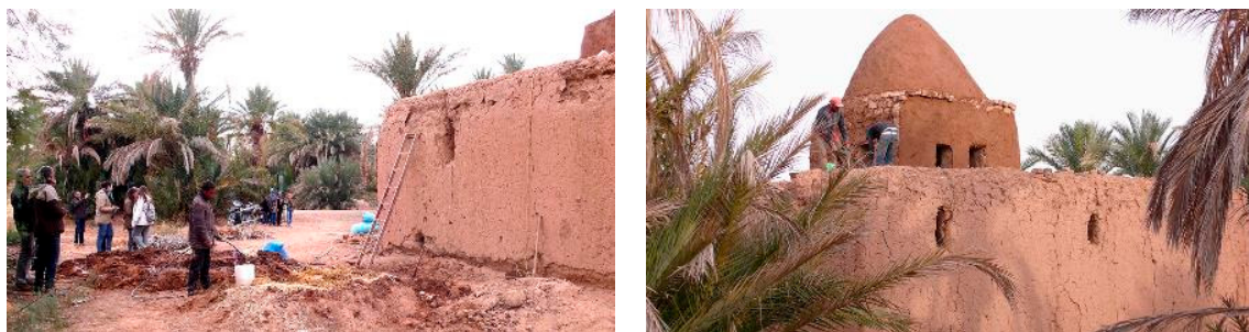
Figure 10. Restoration works of the marabout.
