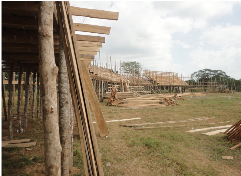
Figure 11. Image of the assembling of a Corraleja , where the main constructive elements are evident. Source: Merwan Chaverra, 2017 [14].
