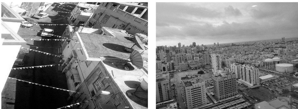
Figure 11. The use of the improper finishing materials for the roofs and building facades.
