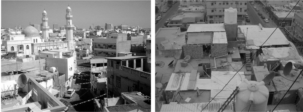
Figure 9. The use of roofs as storage and waste places.
