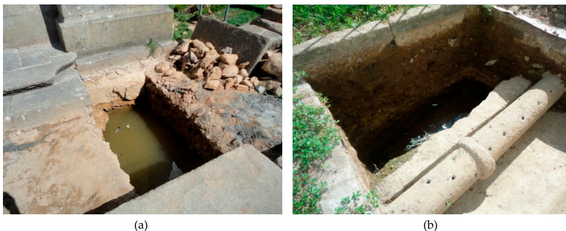
Figure 6. Water table visible in the inspection trenches days after the excavation (summer period). (a) Excavation 1: water level at -0.93 m below the nave floor; (b) Excavation 3: water table at -1.10 m measured from the floor of the nave.
