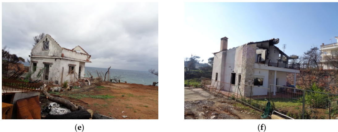
Figure 10. Pictures of buildings characterized as repairable (a–c), non-repairable (d,e), or with a nonrepairable upper floor (f).
