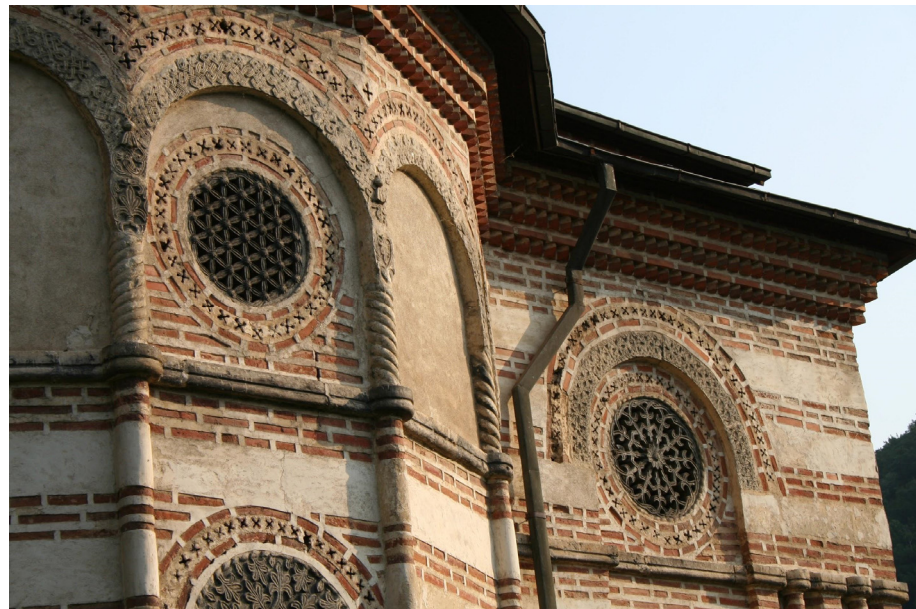
Figure 14. Exterior view of the upper portion of the church, showing the plastered and painted surfaces under the arches, Cozia Monastery, Wallachia, modern-day Romania (source: Elisabeta Negrău).
