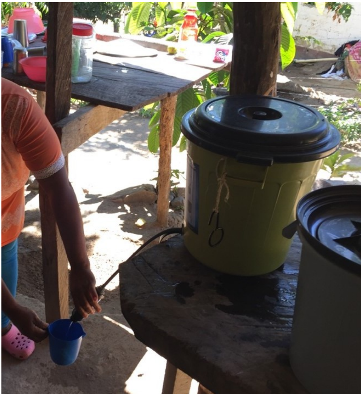
Figure 1. Installed water filter in a remote village inhabited by the Wiwas.
