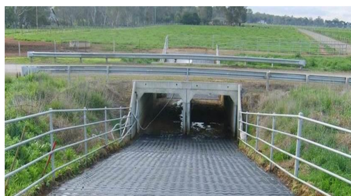
Figure 2. An example of an underpass in Victoria, Australia.
