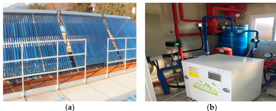
**Figure 2.** Heating systems used in the experiment. (a) Evacuated tube collector. (b) Geothermal heat pump system with circulating pipes and water storage tank.
