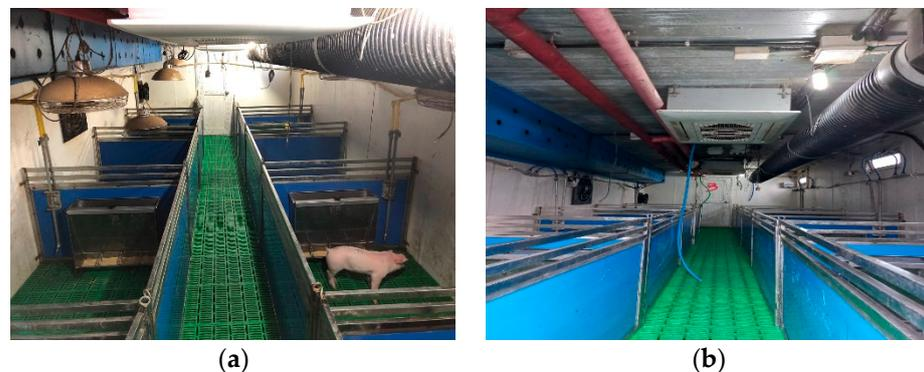
**Figure 1.** Inside pictures of pig houses used in this study. (a) Control house with heating lamps of adjustable height. (b) Pig house installed with GHPS heating system.
