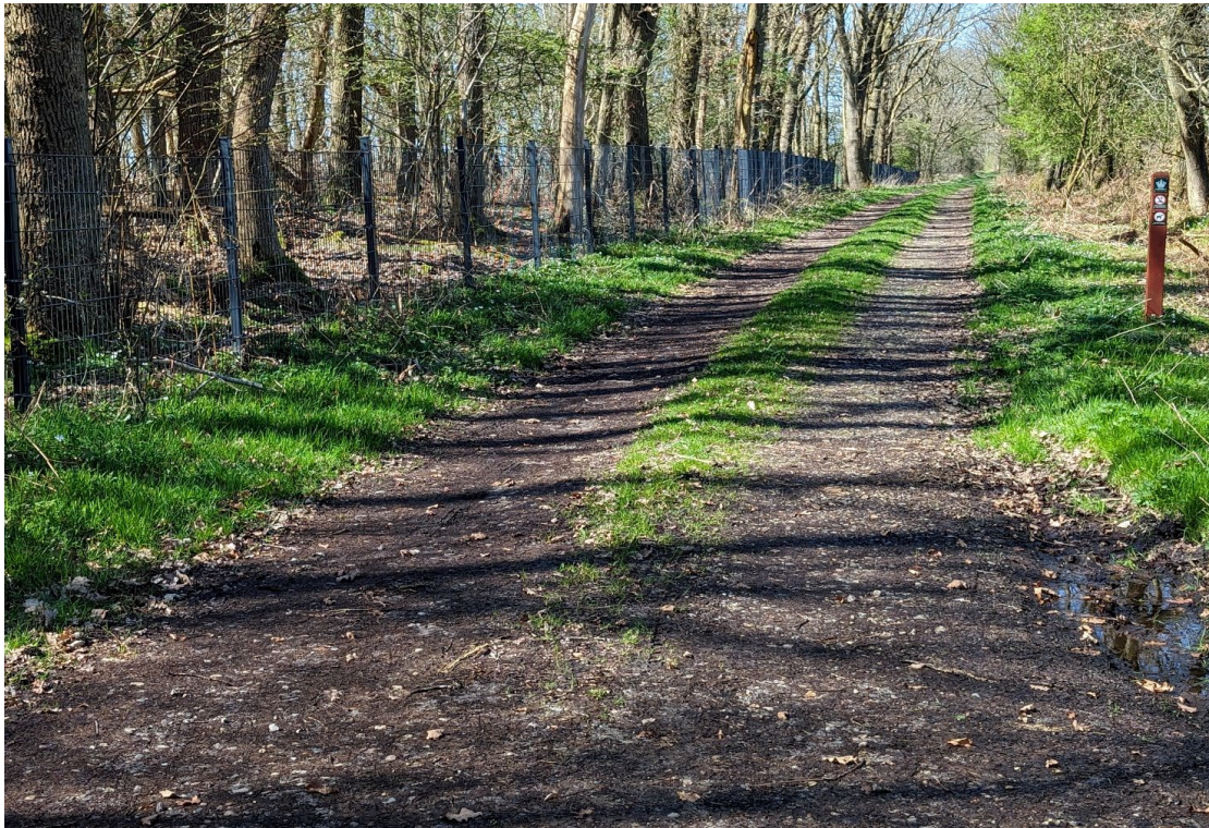
Figure 1. The wild boar fence between Denmark and Germany. The fence is 1.5 m high and has been dug 0.5 m into the ground (photo courtesy of Dr. Gordon Spronk).
