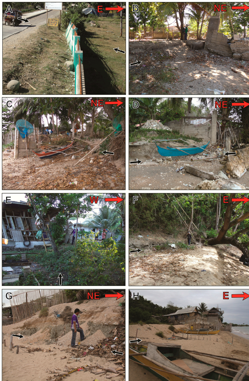
Figure 7. Damage caused by the ground rupture to structures and vegetation. (A). The unrepaired fence in McKinley, Guihulngan shows left-lateral offset due to the ground rupture. (B). Breaking and tilting of a concrete structure south of Guihulngan town proper due to vertical displacement and horizontal shortening caused by the ground rupture with simple-flexural-fold scarp. (C). Breakage of concrete fence in McKinley, Guihulngan. The ground rupture which consists of a simple scarp followed a pre-existing terrace scarp and caused ~ 1m vertical separation. (D). A similar but smaller ground rupture scarp in Basak, Guihulngan also damaged a fence. (E). Concrete structure was deformed and offset by the ground rupture in Bgy. Padre Zamora, Guihulngan. A 0.7 m scarp face is exposed but the larger part of vertical separation is caused by warping, which in turn caused the tilting of trees. (F). The scarp in McKinley, Guihulngan also caused the tilting and collapse of a tree. (G). 1–2 m of scarp along the ground rupture in McKinley, Guihulngan. The scarp cut unconsolidated calcareous sediments overlying a gray sandstone layer. (H). The development of a pressure ridge on the upthrown side of the scarp located directly to the south of (G) caused the tilting of structures.
