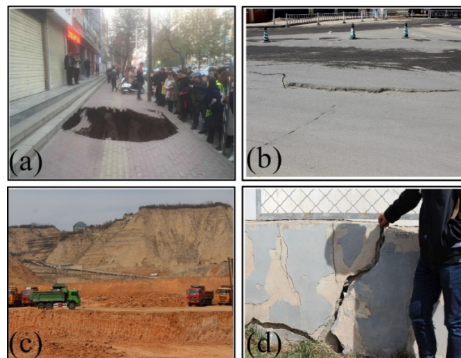
Figure 1. Surface deformation observed in Lanzhou. (a) ground collapses, (b) road ground sinks, (c) creating new land areas by cutting through the mountains and (d) cracks and openings in the wall.
