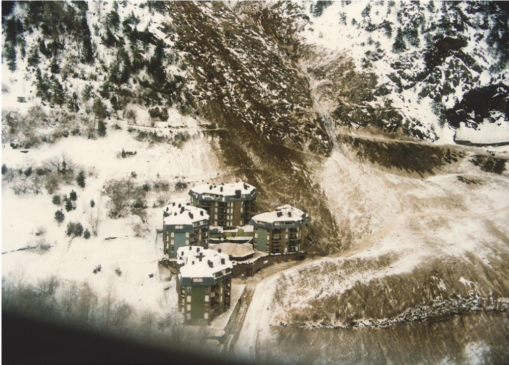
Figure S5. Helicopter view of the Les Fonts d'Arinsal avalanche run-out zone. Detail of Prat Sobirans buildings.
