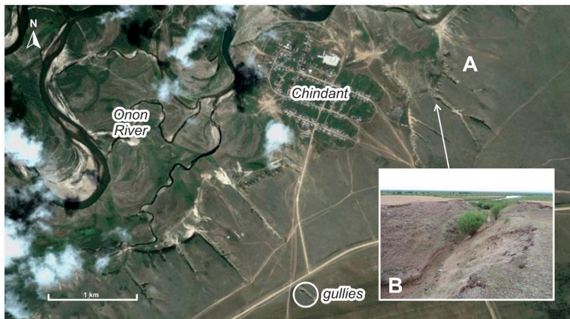
Figure 7. Stretch of the Onon river valley. Coordinates: 50033'44.29" N; 115023'32.13" E. The terrace cut with gullies (A). The image was taken on 8 March 2019. (B) Image of the gully (taken on 16 August 2015), its location is shown with the arrow.
