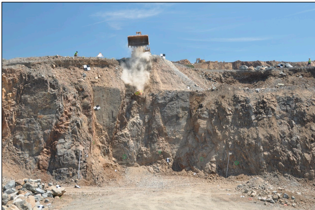
Figure 3. Picture of a block falling down in test site 3.
