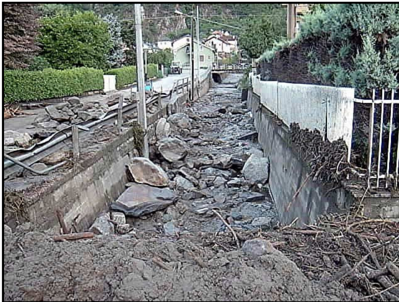
Figure 2. Debris flow deposit in channel bed.
