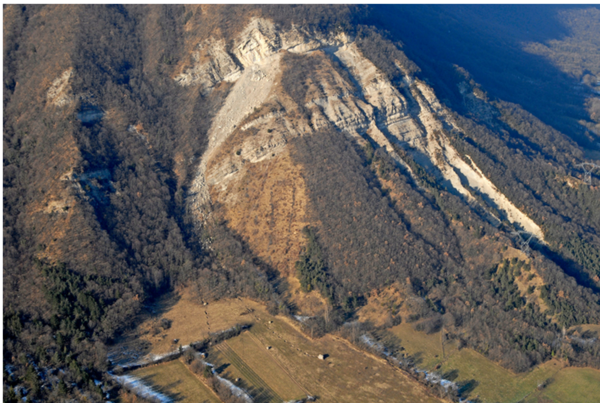
Figure 1. Rockfall with a volume bigger than 1000 m 3 occurred in 2008 in Saint-Paul de Varcès (French Subalpine Ranges). Note steep talus slope and large boulder runouts. Photo S. Gominet (IRMa).
