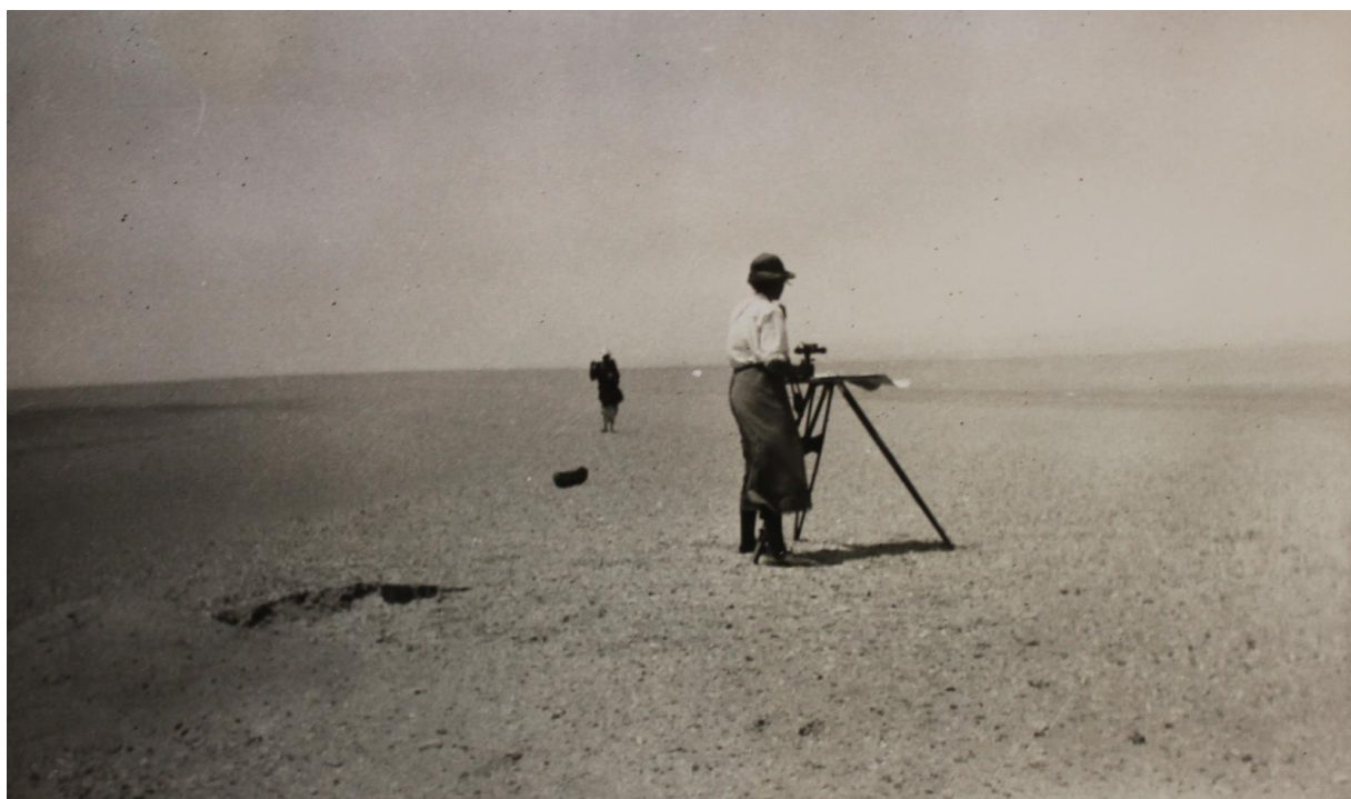
Figure 4. Fayum. Elinor Wight Gardner conducting a survey of the concession area between Kom Ashim and Qasr-es-Sagha to generate a contoured map. Associated note by Caton Thompson reads “High mid. day winds and dust were often a trouble.” Image courtesy of UCL Special Collections.
