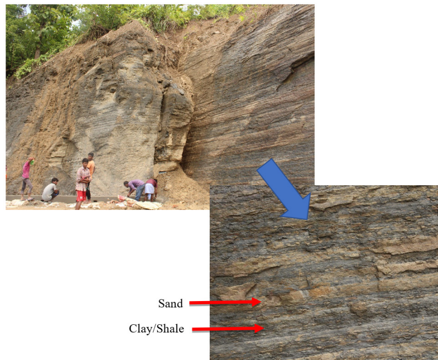
Figure 5. Different layers of soils at Shapchari Shal Bagan located in the landslide areas.
