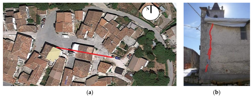
Figure 15. St. George church in Terracino (Accumoli): (a) aerial photography (adapted from Google Maps) with east–west axis orientation (red line); (b) façade overturning mechanism (cracks emphasized in red).
