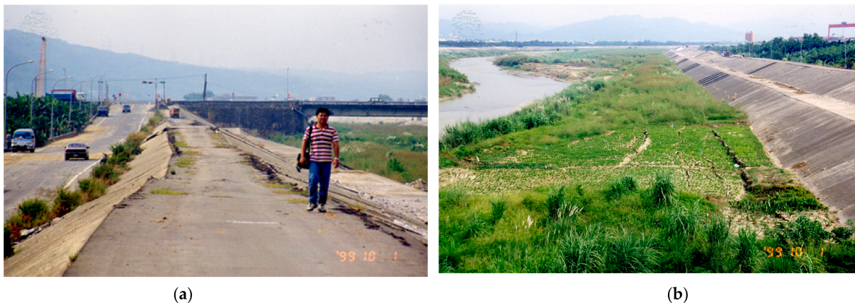
Figure 12. Damage of the demonstration site after 1999 Chi-Chi Earthquake, (a) settlement of the embankment, (b) lateral spread of floodplain.
