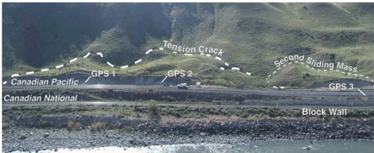
Figure 2. Ripley slide geometry including CN and CP railways and installed GPS on the site.
