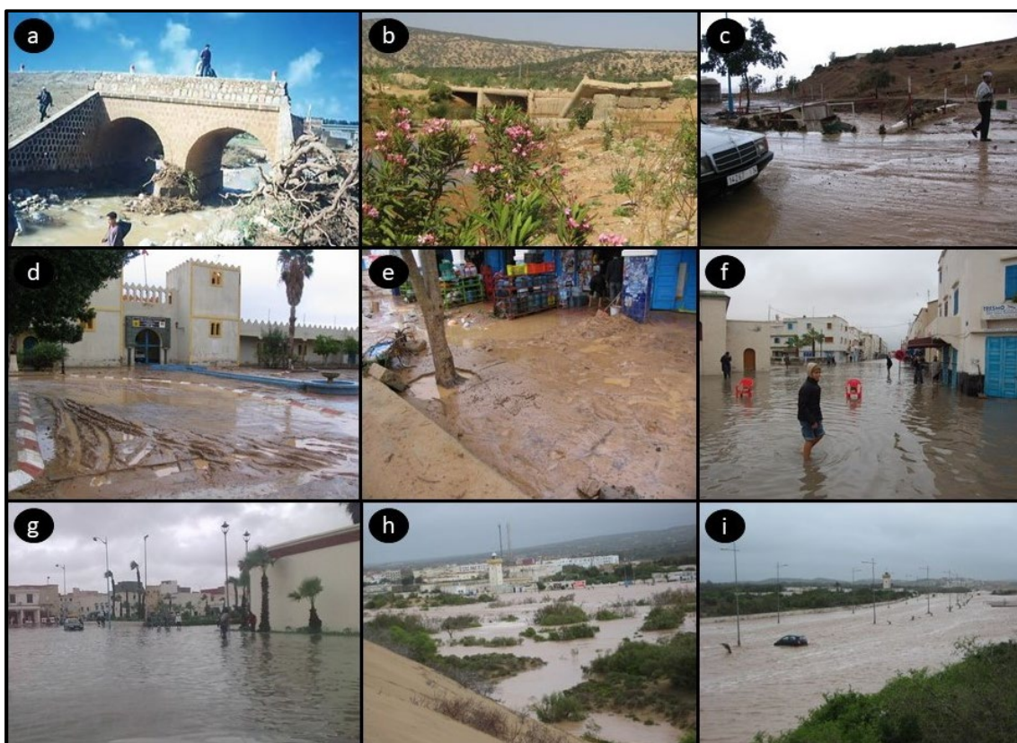
Figure 5. Damages to the infrastructures of the Essaouira province: (a) destroyed bridge of Smimou Village during the 1996 floods; (b) collapse of the existing bridge upstream of the village of Tafedna damaged by a previous flood in 2002; (c) flood of the Oued Tamarar on the 25 October 2006; (d) the traces of the floods of the Tamarar center on 25 October 2006; (e) the traces of the floods of some shops in center of Tamarar on 25 October 2006; (f) Hay and Mosque Lalla Amina during the floods of 24/25 December 2009; (g) state of the boulevard Lalla Aicha and the place Bab Marrakech during the floods of 24/25 December 2009; (h) and (i) overflow of the Oued Ksob in the city during the floods of 24/25 December 2009.
