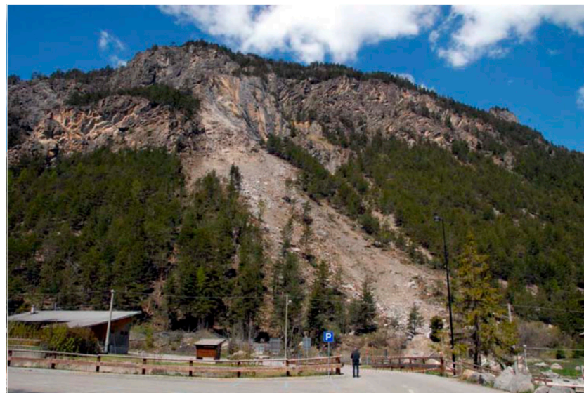
Figure 3. View of the examined rock slope [18].
