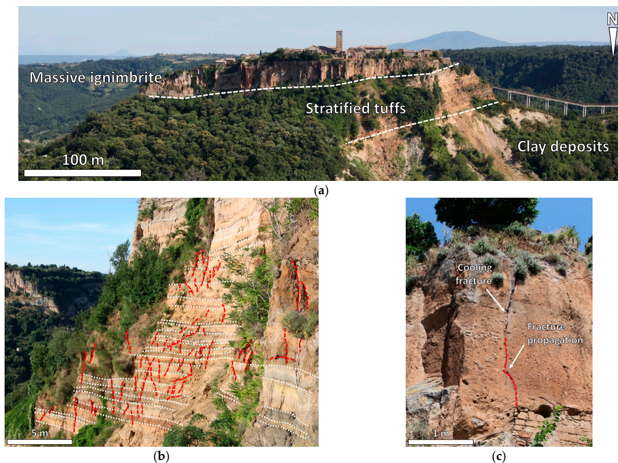
Figure 10. Rock mass and slope damage at Civita di Bagnoregio: (a) View of the volcanic plateau. Note the varying behavior of the materials that characterize the area, particularly the landslide developing in the clayey deposit. White, dashed lines mark the boundaries between the different materials. (b) Slope damage features (dashed red curves) affecting the stratified tuff, inducing a decrease in the overall rock mass quality that, in turn, affects the failure and deformation behavior of the slope. (c) Brittle damage, in the form of a fracture propagation from the tip of a cooling fracture, in the massive ignimbrite.
