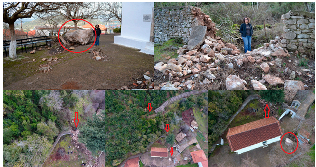
Figure 9. Pictures taken from Platiana region after rockfall event.
