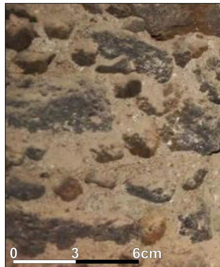
Figure 2. Masonry of the bell tower: photo of the internal side.
