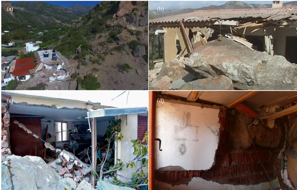
Figure 1. Examples of rockfall damage for buildings (a) collapse of a touristic apartment in Ierapetra, Crete, Greece. (b) Wall damage in Alyki, Voitia, Greece. (c) Residences hit by rockfalls in Mytilene, Greece. (d) A rock block impacting a wall in Clua, Pyrenees, Spain.
