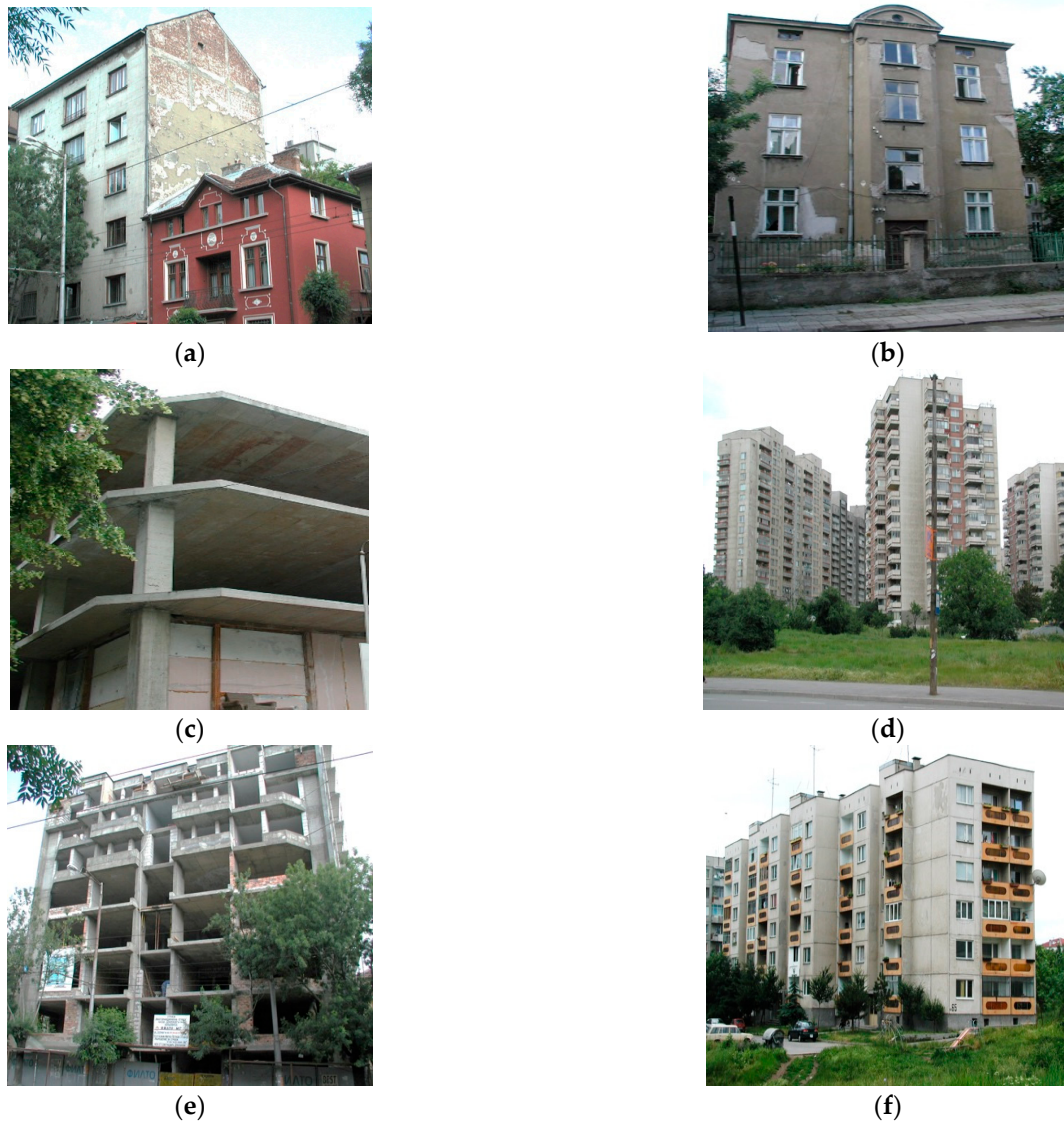
Figure 7. Building typologies in Sofia: (a) five-story masonry building with reinforced concrete belts, type M1; (b) three-story masonry house with wooden beams, type M2; (c) skeletal beamless reinforced concrete structure, type RC2; (d) structures with reinforced concrete shear walls, type RC4; (e) reinforced concrete structure with shear walls and columns, type RC5; and (f) six-story large-panel building, type RCp7.
