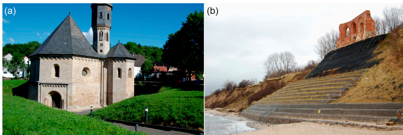
Figure 5. Evidence of extreme atmospheric events affecting historical building and objects of cultural heritage. (a) Chapel in Grünsfeld (central Germany) was built on a floodplain, but is now located several metres below the ground level in the vicinity due to many episodes of flood deposition and floodplain build-up over centuries; (b) cliff undercutting by severe storms caused its considerable retreat since late medieval times and, finally, nearly complete destruction of a late 15th century church in Trzęsacz (NW Poland) (all photos by P. Migoń).
