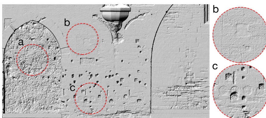
Figure 6. Raster hillshade 315° azimuth 45°: (a) surface roughness not visible from photographs, (b) surface roughness not visible to the naked eye, and (c) carved symbols, barely visible on site.
