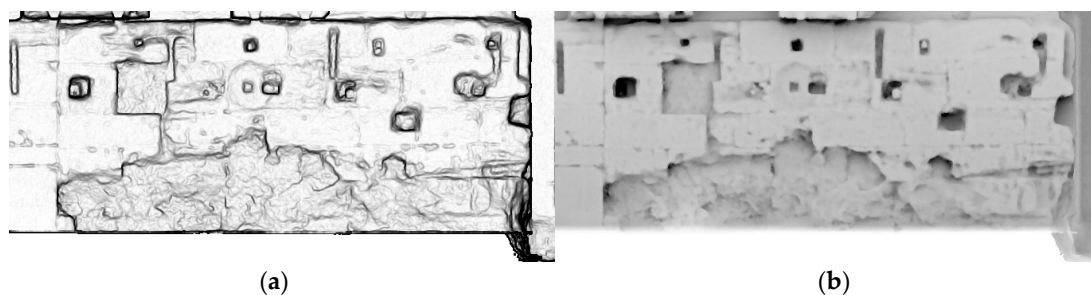
Figure 8. Deterioration of the stone: (a) the boundaries between surfaces, the slope, is identified; and (b) the sandstone is identified as well as the disintegration of the stone (ambient occlusion).
