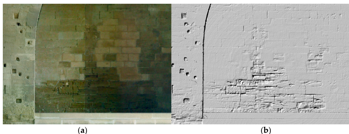
Figure 9. Identification of previous interventions with different stone: (a) RGB left; and (b) disintegration of stone (hillshade).
