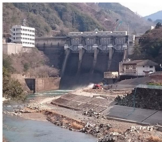
Figure 3. Kanogawa Dam and its management office (left).
