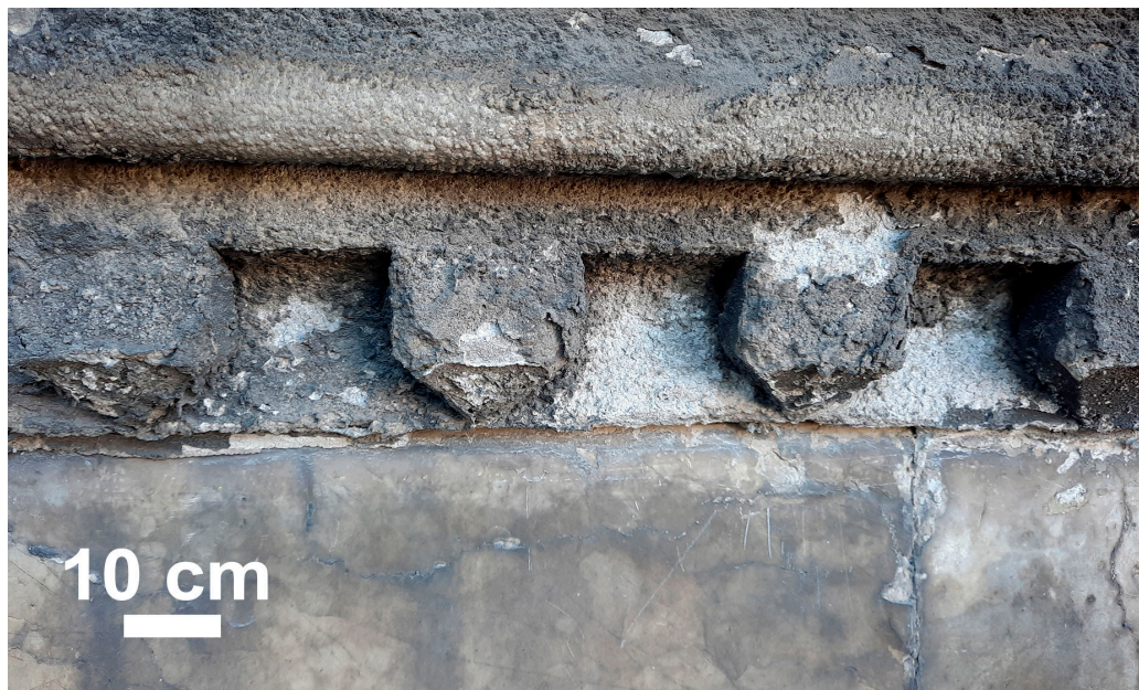
Figure 1. Architectural element (artificial stone) affected by black crust (laminar), together with blistering phenomena. Blistering is evidenced by the lack of black crusts in some areas. Image from the Monumental Cemetery of Milan (Italy).
