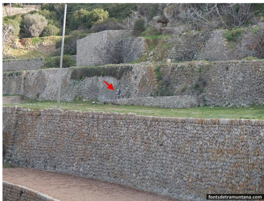
Figure 21. Font de sa Basseta, a spring-flow tunnel located in Banyalbufar in a stepped terrain area. The red arrow indicates its outflow point. Reproduced from sites.google.com/view/fontsdetramuntana (accessed on 6 December 2023). Photo credit: Andreu Morell.
