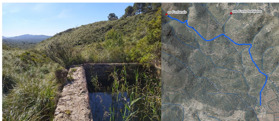
Figure 17. Es Fontanals spring (Left) and its channel, now in ruins (Right). Photo credit: P.F. Castro. Orthophoto (2021 flight) from IDEIB (Infraestructura de Dades Espacials de les Illes Balears).
