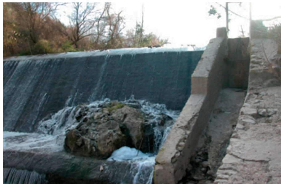
Figure 8. Downstream of the El Cerrajón weir and diversion channel of the ecological flow (source: Technical documentation of the set of waterwheels, watermills and river mills in the province of Cordoba [69]).
