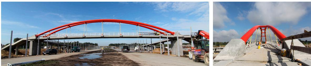
**Figure 1.** Side and front view of the arch footbridge above expressway S8.
