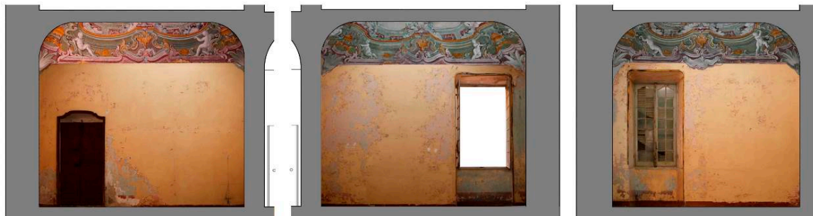
Figure 8. Survey carried out for the first room.
