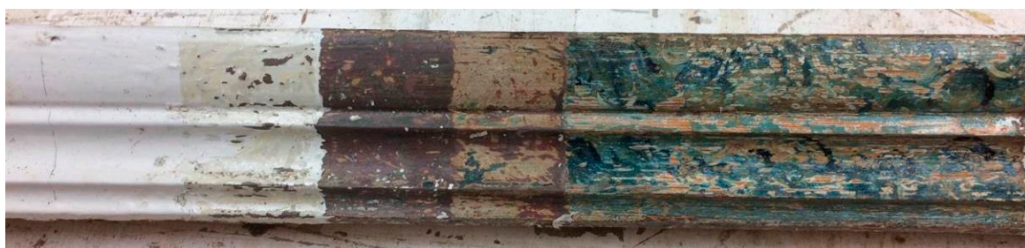
Figure 15. Stratigraphical analysis of the wooden moldings (entrance door, first room).
