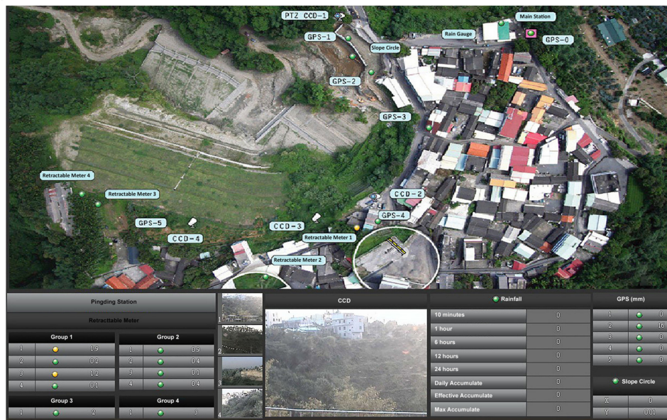
Figure 10. Integrated monitoring data display.
