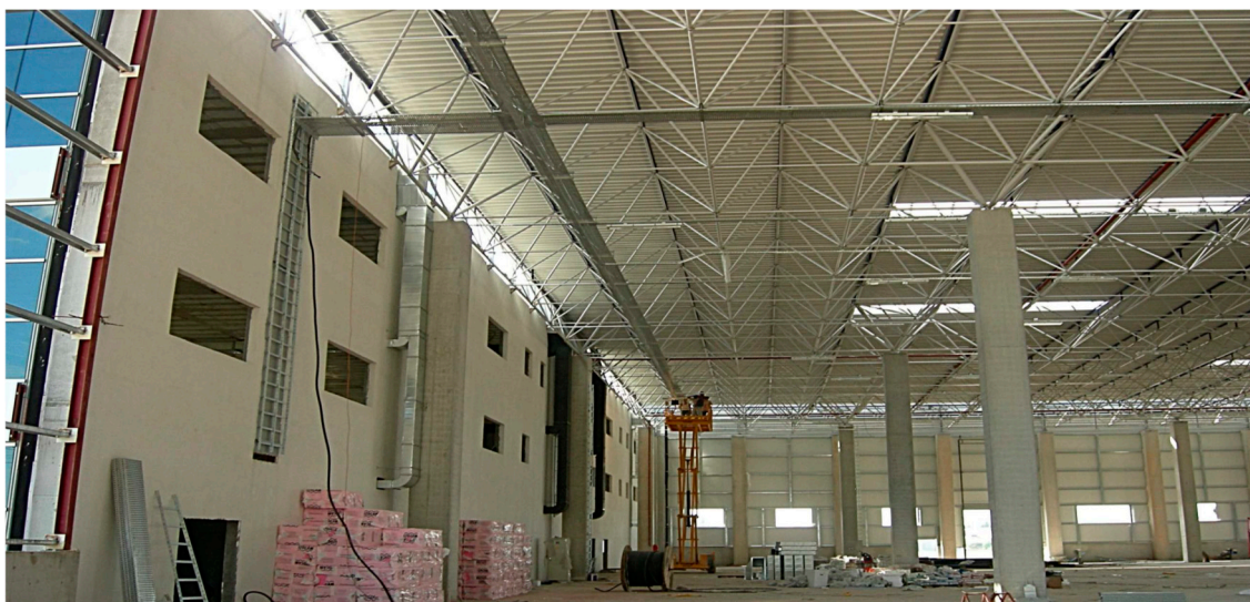
Figure 3. Overview of the roof structure.
