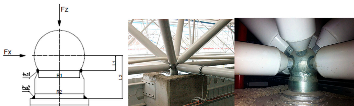
Figure 5. View of the spherical joints and the supports.
