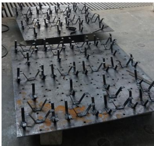
(a) Line welding for the one end of CSCs
