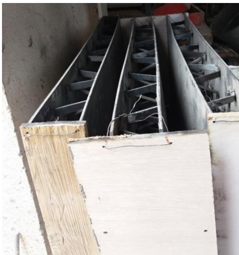
(a) Concrete moulding
