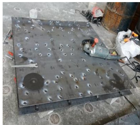
(b) Plug welding for the other end of CSCs
