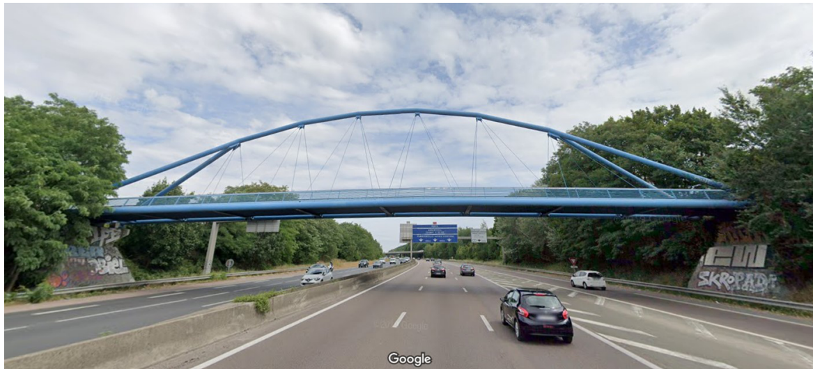
Figure 28. Montigny-Les-Cormeilles footbridge, France. Photo: Google Maps, Street View.
