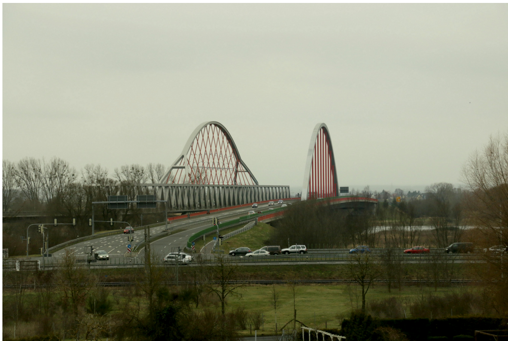
Figure 4. Wittenberg Bridge over the Elbe River. Left: Forked railway tied-arch bridge with two sets of lateral hangers. Right: Road bridge with single central set of hangers. Photo: Michael Fiegle. Wikimedia Commons.
