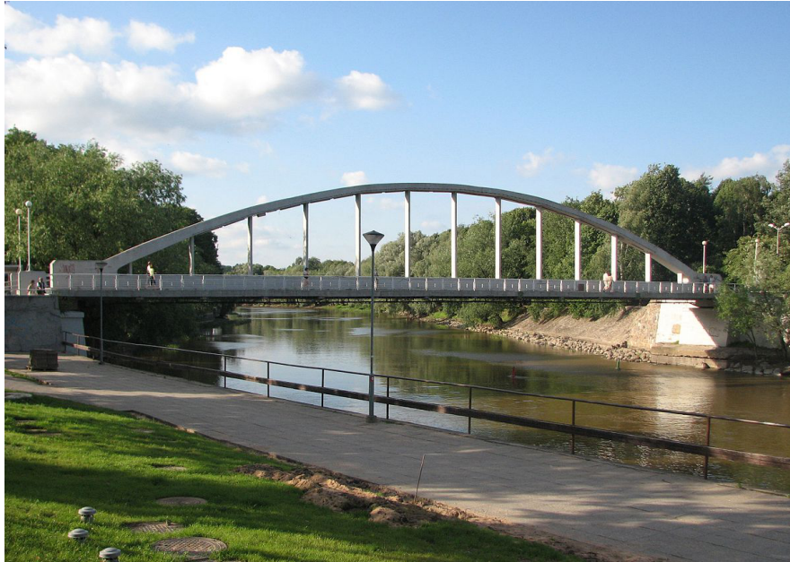
Figure 2. Tied-arch bridge in Tartu over the Emajõgi river (Estonia). Photo: HendrixEesti, Wikimedia Commons.
