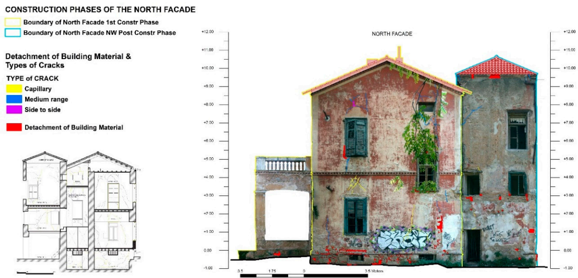
Figure 13. Thematic map of cracks and detachment of building materials depicted on the north façade of the building.
