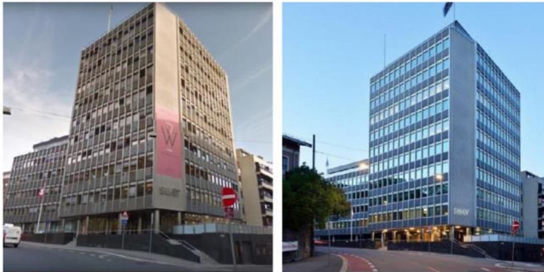
Figure 14. The Wergelandsveien 7 building in Oslo before (left) and after renovation (right) [10].
