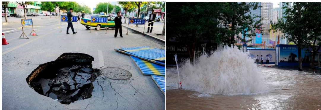
Figure 1. Pavement collapse and pipe burst caused by cracks in concrete pipes.
