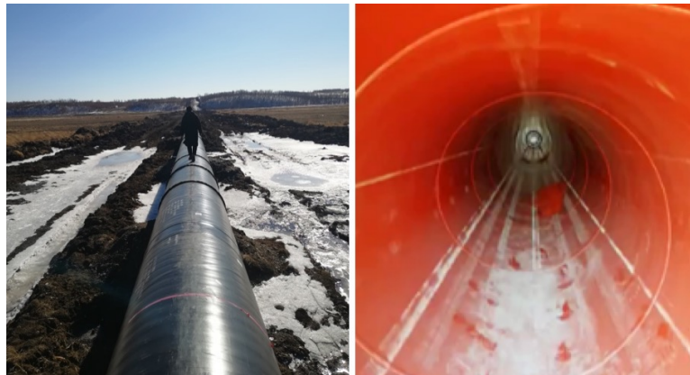
Figure 12. Testing scene at the Heihe Pipeline Construction Site.
