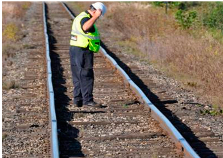
Figure 4. Manual joint inspection by a technician in the field.
